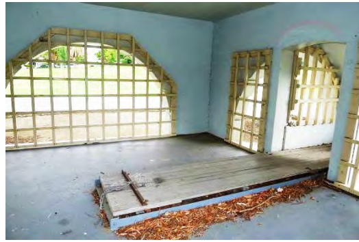
Figure 3.21: Undercroft area, showing boarded drawbridge and tracks.
