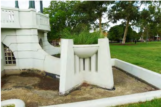
Figure 3.15: Typical detail of rotunda base and fern bowls within basin.
