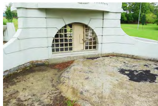
Figure 3.19: Basin and access door to undercroft. Note dark-coloured remnants of possibly original asphalt.
