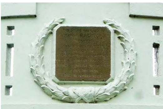
Figure 3.18: Typical trachyte plaque located at the centre of the perforated balustrade on the western side. Similar plaques are located on the eastern and /southern sides.
