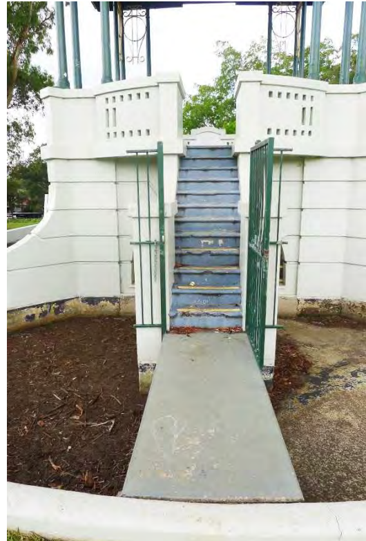
Figure 3.16: Concrete drawbridge and entry stairs into rotunda on northern side.
