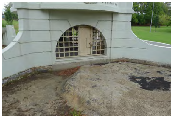
Figure 6.4: Lattice screens and entry door into undercroft.
